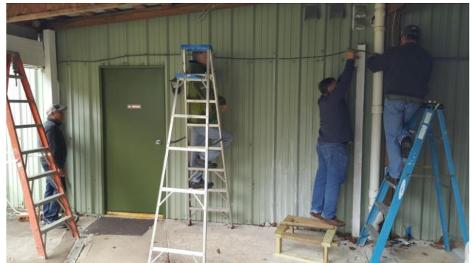
Sam Fontanez, Sal Fazzino, Jesse Stone & Tom Baker reconfiguring propane lines for the back-up communications generator
